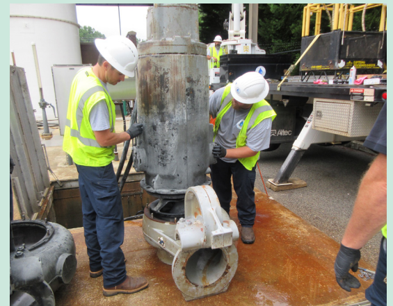
Robert Sims and Josh Dominey pull pumps at the Upper Walnut Creek Pump Station during preventive maintenance. This type of work will be featured during the summer internships being offered by the Authority and SCTC.
